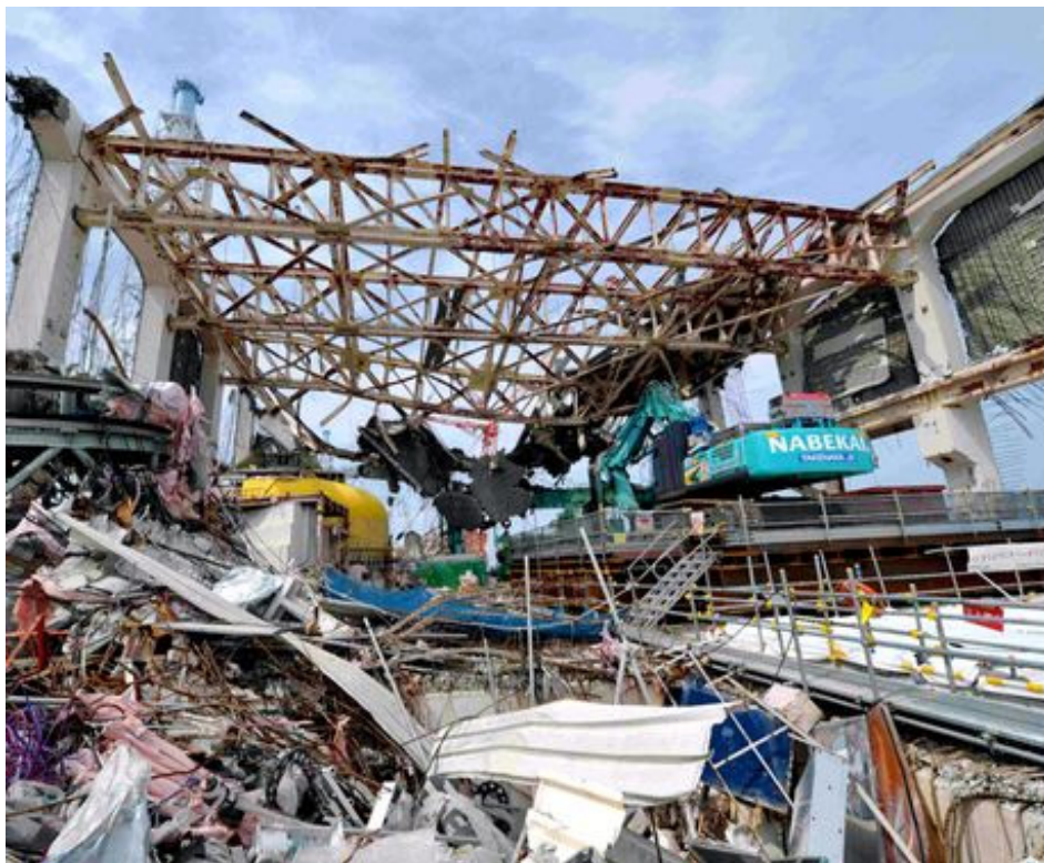
The fifth floor of the No. 4 reactor building at the Fukushima No.1 nuclear power plant as seen on May 26. The spent fuel rod pool is on the right, covered with a white tarp. (Pool)
